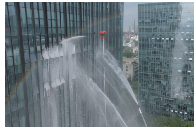
50 Fire hoses - mooring height test 120 meters above ground
