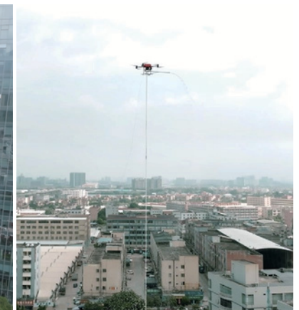
40 Fire hose - mooring height test 170 meters above ground
